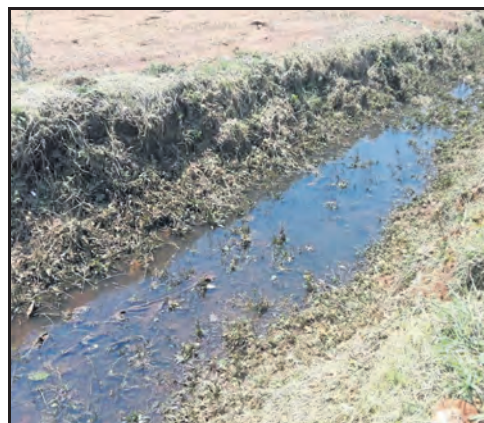
The trench in Risiville is fast getting clogged again as a result of residents' illegal dumping.
